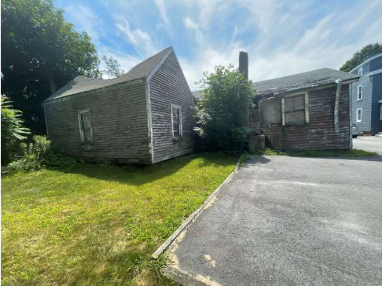
Accessory Building (Rear View)
