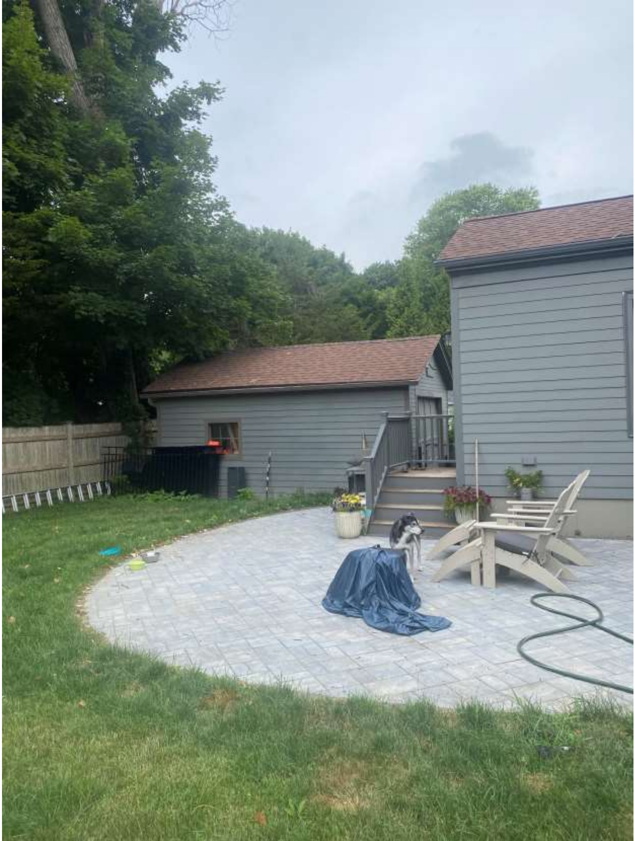
Rear Yard / Garage View
